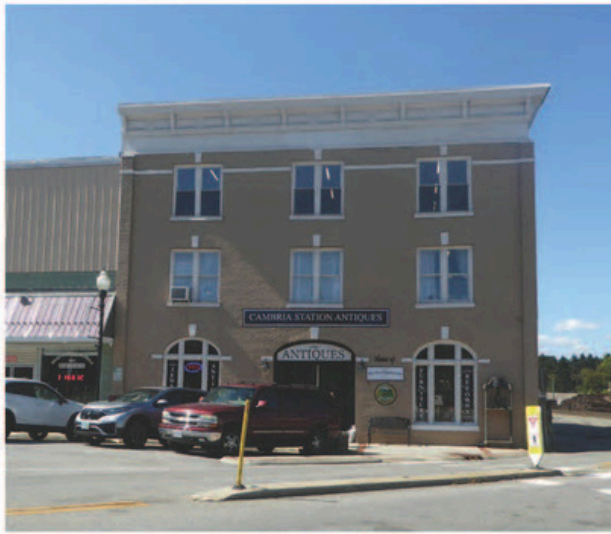
Cambria Station Antiques is in a 3-story building that once served as a storage facility for goods that arrived by train.
