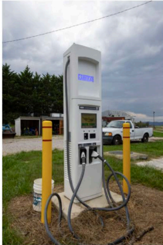
An interesting and forward-thinking amenity at the airport is a charger for BETA Technologies electric aircraft, which Holt says have visited the airport
